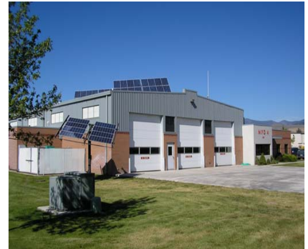
Missoula Fire Department Station #4 Photovoltaic Panels
