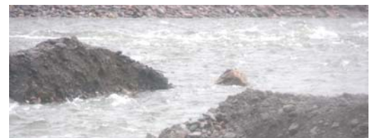
Flow into the new channel increases; By late Friday, about 20% of the river flow was in the new channel (as projected). By Monday, about 70% of the river flow had been diverted into the new river channel at the base of the bluff.
